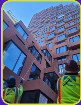
The team working on The Canyon
